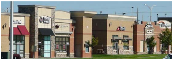
In the image at left, masonry elements are visually supported by other masonry elements; a sill is used to separate stacked materials; and side-by-side materials transition at interior corners.
