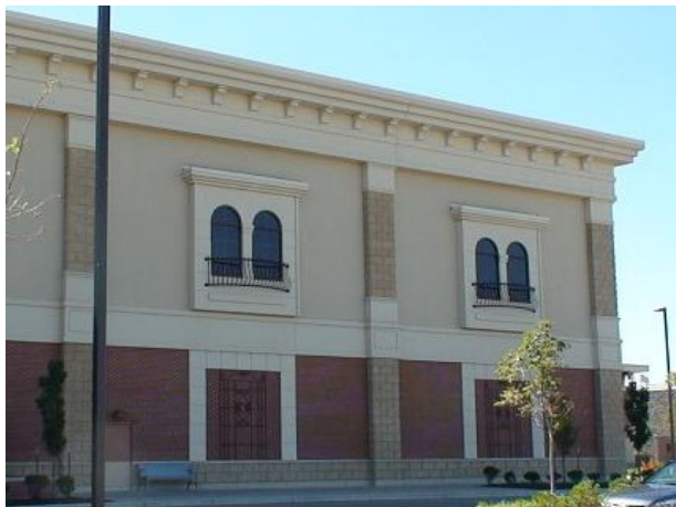
This façade could have been a large blank surface, but instead is broken up by decorative elements that relate to the pedestrian.
