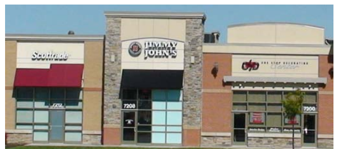
This building's parapet varies in height, and the awnings are not wider than the individual storefronts.
