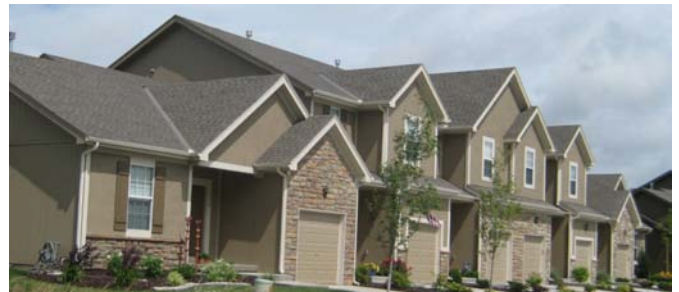
The building above uses a façade reversal, a change in height of masonry material, and a different roof design to create a substantial difference between the two-story units. The building remains unified by similar architectural style, similar building materials, similar window and door patterns, and similar architectural elements.
